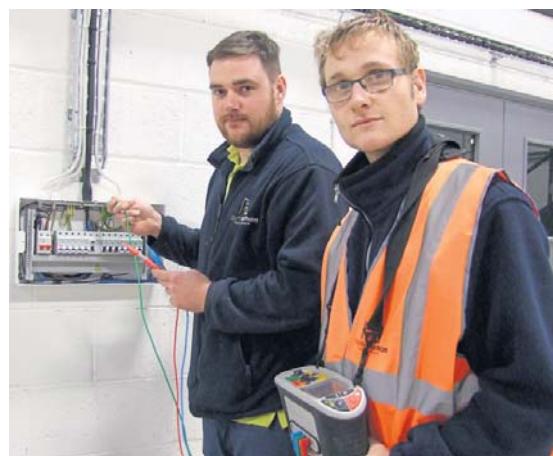
DISC trainee Kryran Harris carries out an insulation test with County Durham Housing Group electrician Joe Hunter
