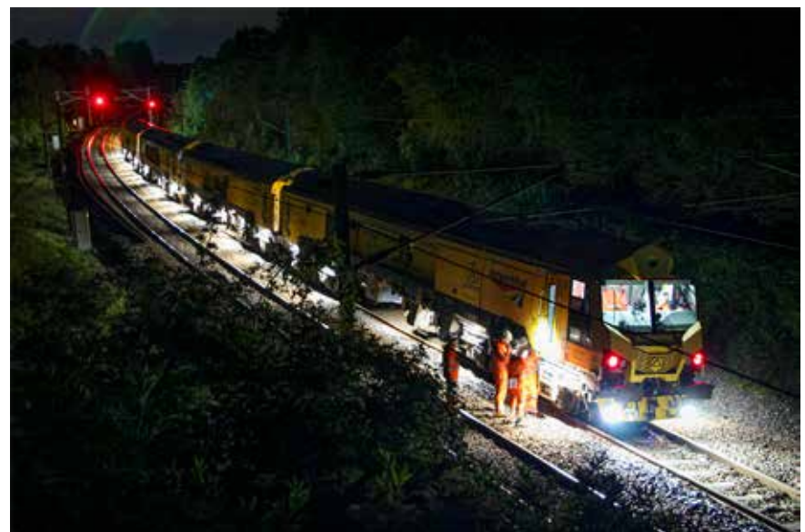
This is a Rail Milling Machine, which was in operation in the early hours of a Sunday morning. The photo was taken on Lime Lane, just next to Ashcourt, near Aycliffe Village. As far as I am aware, it was carrying out routine maintenance and works by taking a small layer of metal off the top of the rail to remove any small defects.
